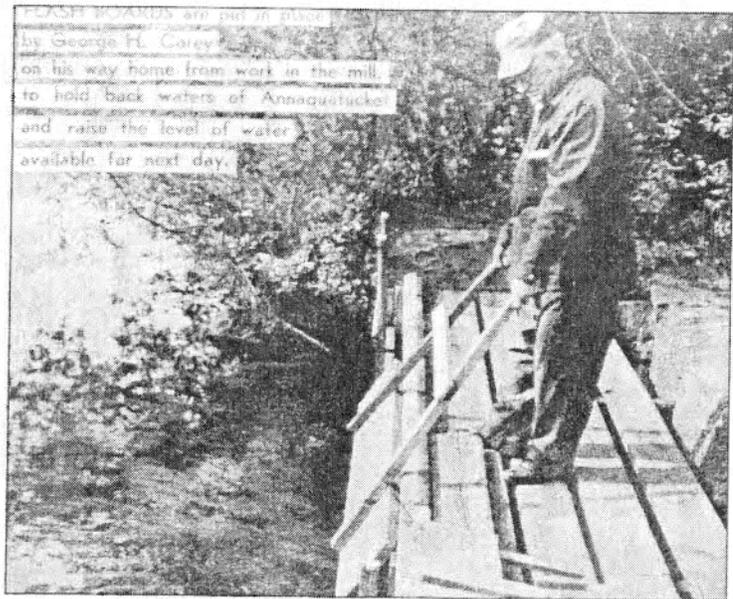
FLASH BOARDS are put in place by George H. Corey on his way home from work in the mill, to hold back waters of Annaquatucket and raise the level of water available for next day.
